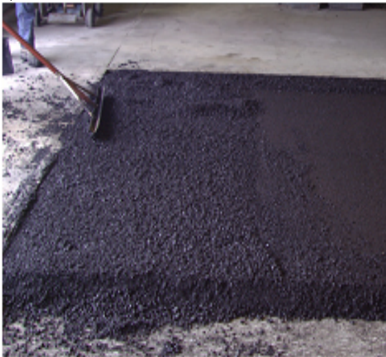
Installing Test Mix
