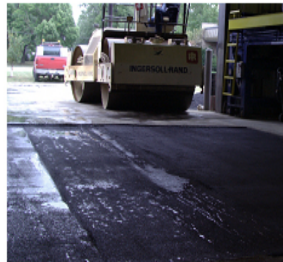
Compacting Test Mix
