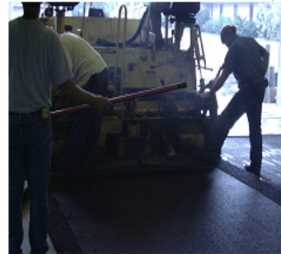
Compacting Test Mix
