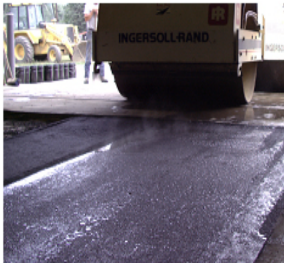
Compacting Test Mix
