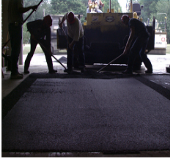
Compacting Test Mix
